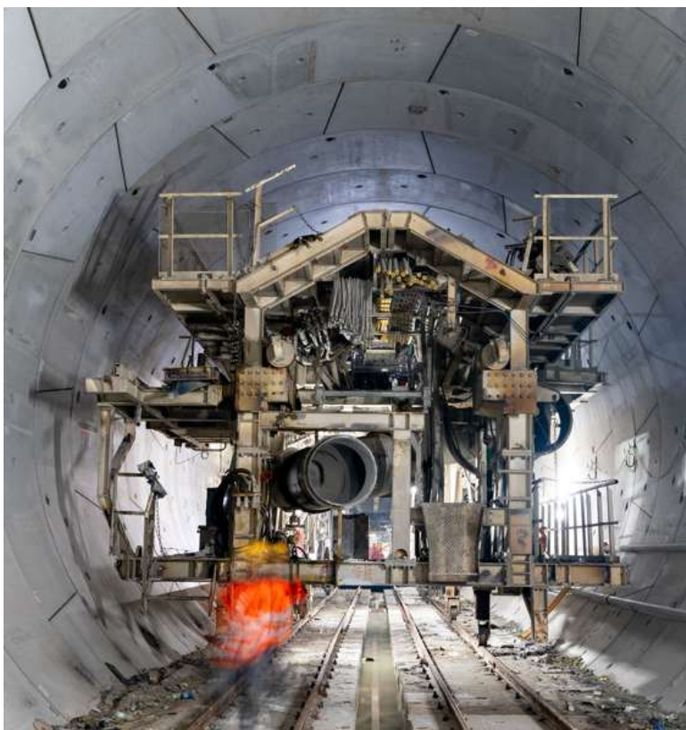
H61 Mules – excavation of main tunnels completed
