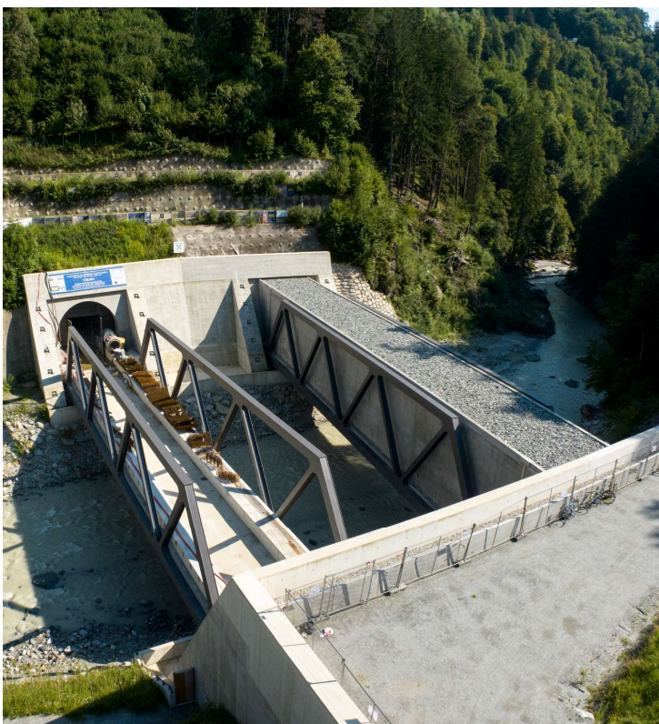
H21 Sill gorge - completed
