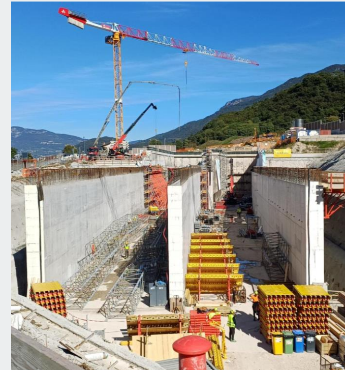
Construction of Artificial Tunnel
