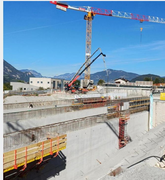
Construction of Artificial Tunnel
